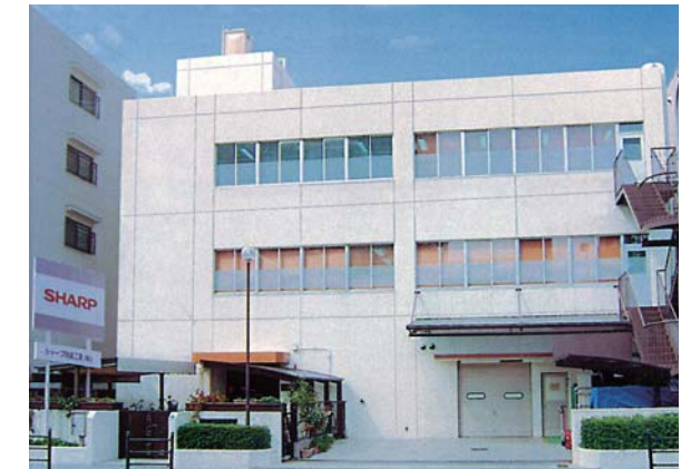
New factory building for the Hayakawa Tokusen Metal Limited Partnership, completed with local support
