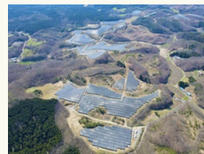
Samegawa Aono Solar Power Plant
