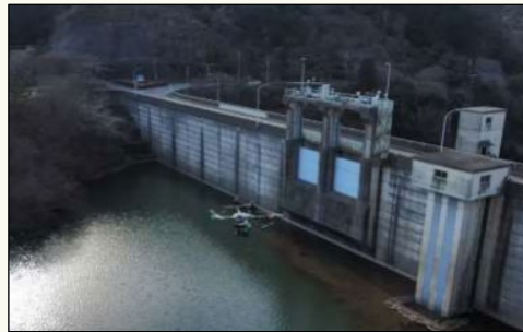
Local 5G validation testing for dam inspection and maintenance
