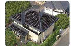
Residential Solar Roof top
