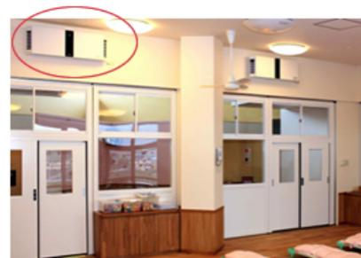
Plasmacluster ion generators installed in a day-care center
