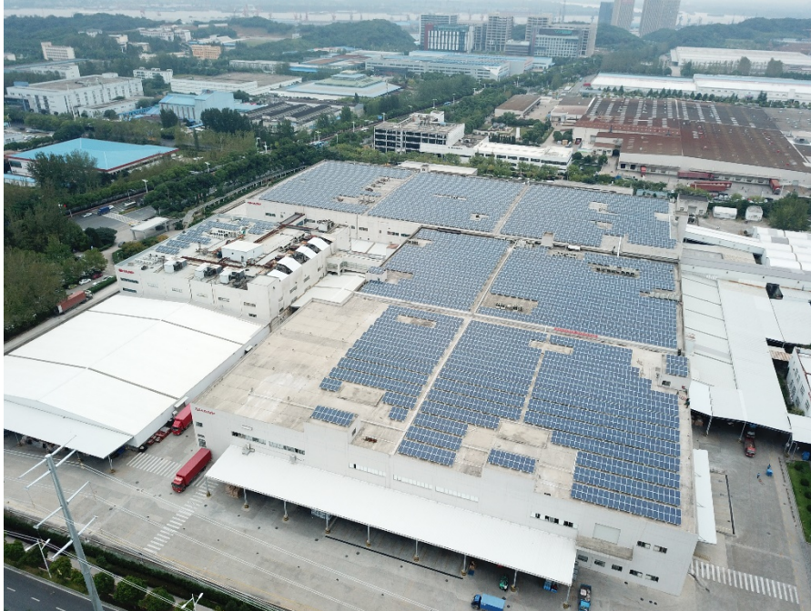
Solar power system installed on the plant roof
