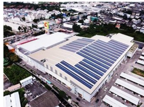
Installation of rooftop solar modules
