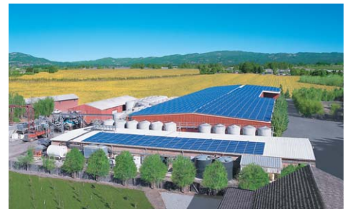
Photovoltaic power generation system introduced at a Californian winery
